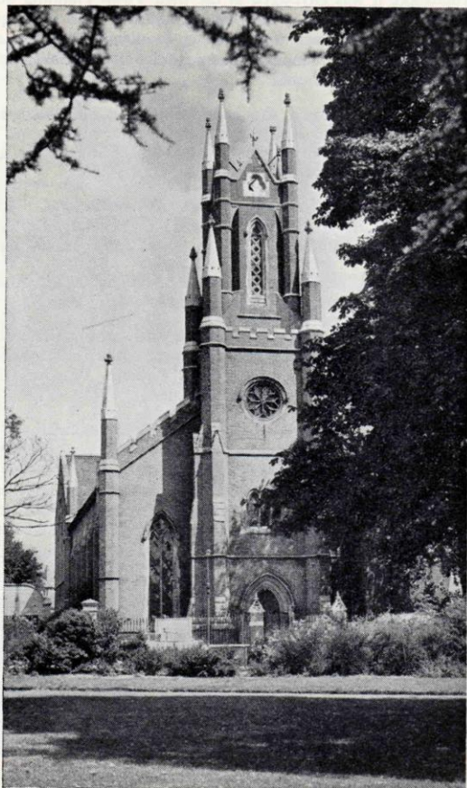
THE UNITED PRESBYTERIAN-CONGREGATIONAL CHURCH BRUNSWICK PLACE, SOUTHAMPTON
